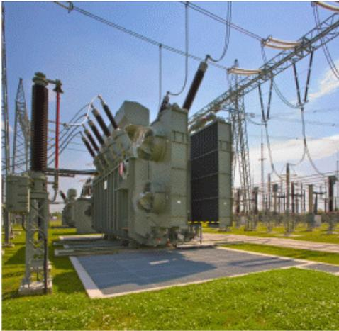
A transformer is a nearly lossless way to convert a high voltage low current condition (high impedance) to or from a low voltage high current condition (low impedance). Watts in equals Watts out. Good transformers are roughly 98 percent efficient! Big ones like this can handle thousands of Watts. A little one like the 3619 or 3636 can only handle power levels used by the squawker in a loudspeaker. They are still 98 percent efficient at transforming
